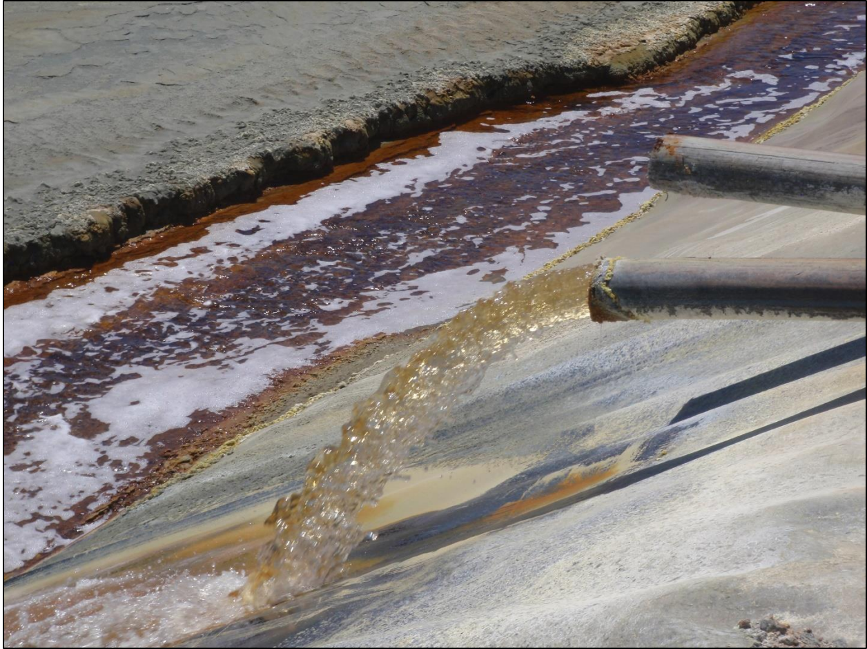
Figure 7b. A mixture of water and tailings is hydraulic discharged behind the Cobre tailings dam at the Atalaya Mining Riotinto copper mine in Spain. The mixture has a solids content of 35% by mass. For the Cascabel Project, the cleaner tailings would have a solids content of 45% by mass, while the rougher tailings would have a solids content of 55% by mass. See long view of hydraulic discharge in Fig. 7a. Photo taken by the author on June 21, 2019.
